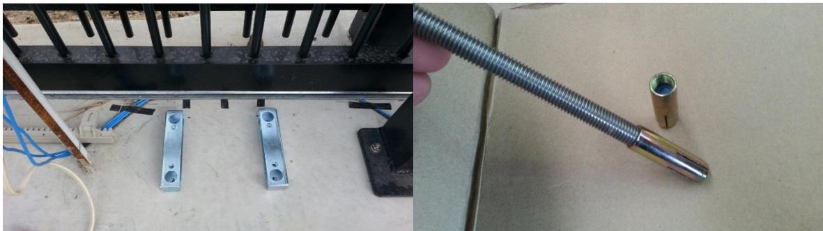
Option 3: If your gate is above 50mm off the ground you can use the mounting plate supplied with the Boxer motor and 4 threaded rods in each corner to act as pylons. The rods have anchor pins that are drilled and hammered/pressed into your concrete pad. Thread the rod into the anchors and place a nut on each rod to the desired height. Place the mounting plate on next, followed by the motor, washers and fasten together with 4 more nuts.
